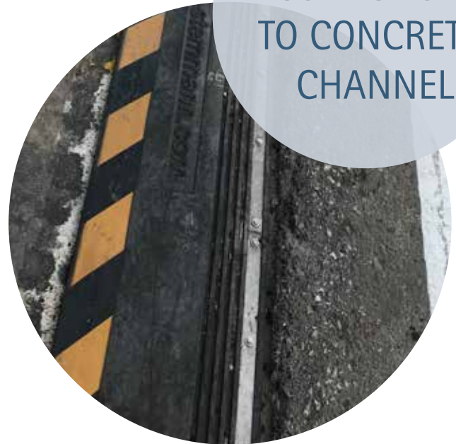
CONCRETE TRENCH WITH BELT FIXING DEVIDE
