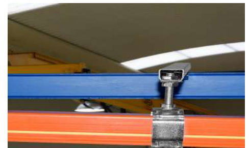
Install the LM-4 line bars at the support points, respecting that the yellow "earth" signal line is always on the same side.
