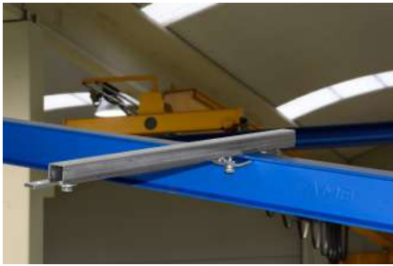
Install universal brackets every 2 or 1.33 meters, according to the assembly scheme
