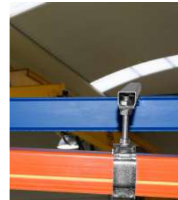
Install the LC-4 line bars at the support points, respecting that the yellow "earth" signal line is always on the same side.
